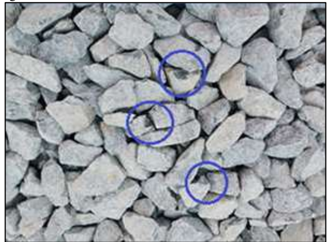
Figure 5: Ballast Particle Damage
